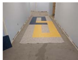
New Tile 1 st Floor Hallway
